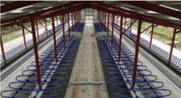
Figure 1: Cow house with a two-row design – an optimum in feed and bed access.
